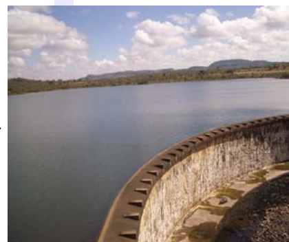
Untapped potential: Zimbabwe is home to some of the best dam infrastructure in Southern Africa
