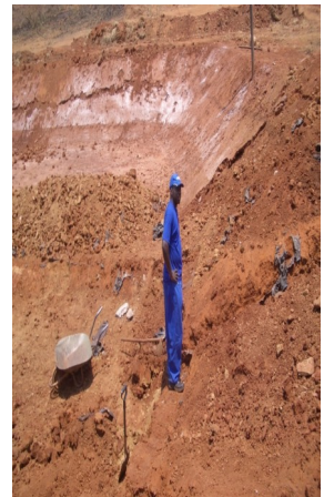
Pond under construction
