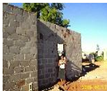
Naomi and her sister are living in a make shift shelter waiting for the completion of their house. Security is their main concern as the area is known to have wild animals roaming around from the near by game park.
