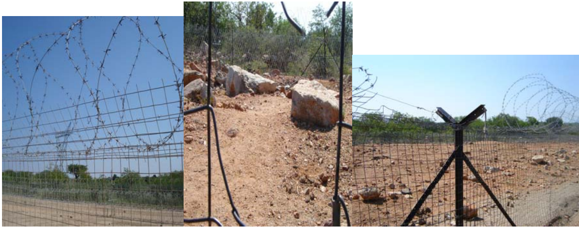
One of three of the seemingly impenetrable border fences (left) and the breach (right)
