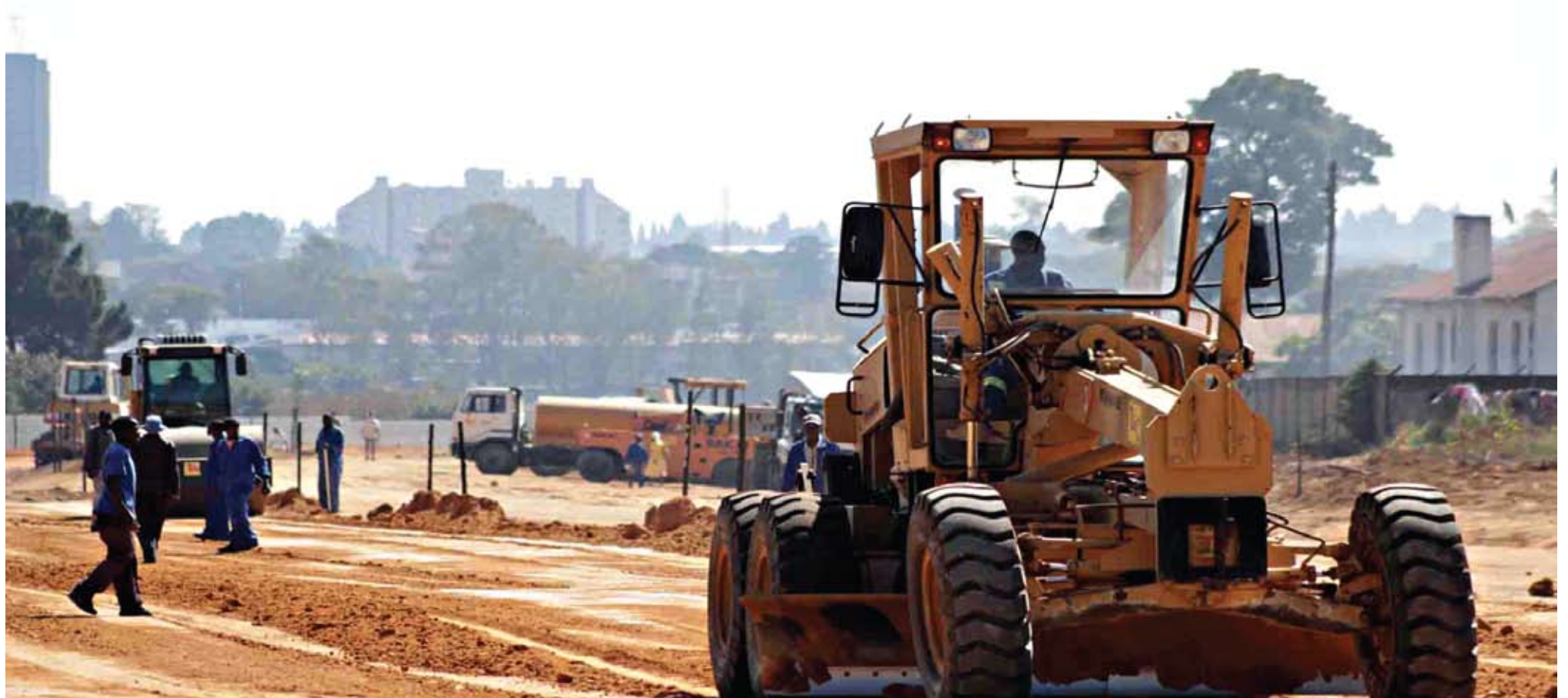
Construction work on site
