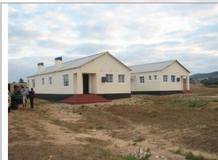
The two completed homes are part of an on going project to construct 13 homes for OVCs.
