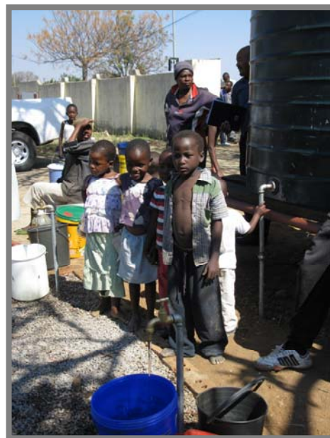
Residents of Mzilikazi suburb collect water from a USAID/OFDA-funded water tank (photo by Johs Pierce, USAID/OFDA).
