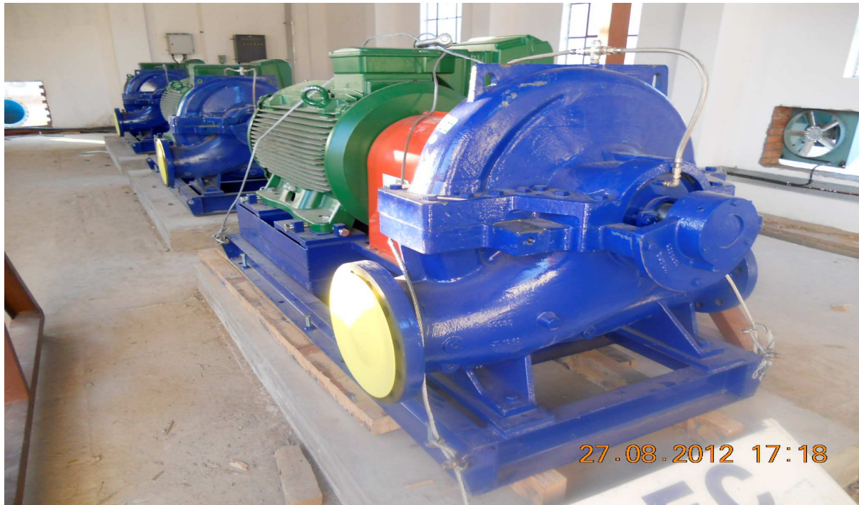
Mtshabezi Pump House
