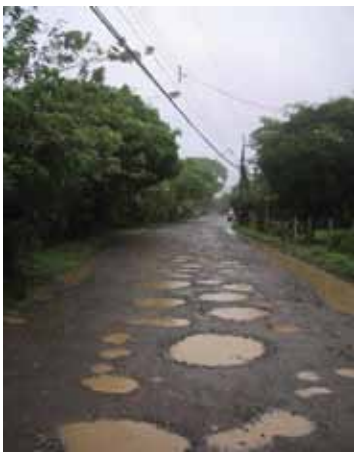
corruption exacerbates poor services- potholes and bad roads
