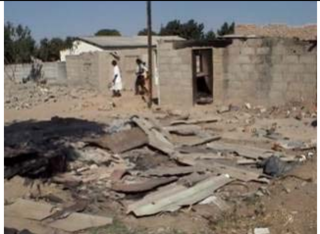
Debris from demolished dwellings, deemed 'illegal'.
