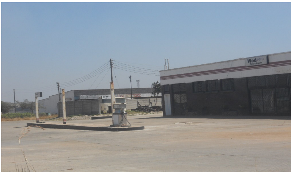
A disused Wedzera Service Station in the Chitungwiza Industrial area.
