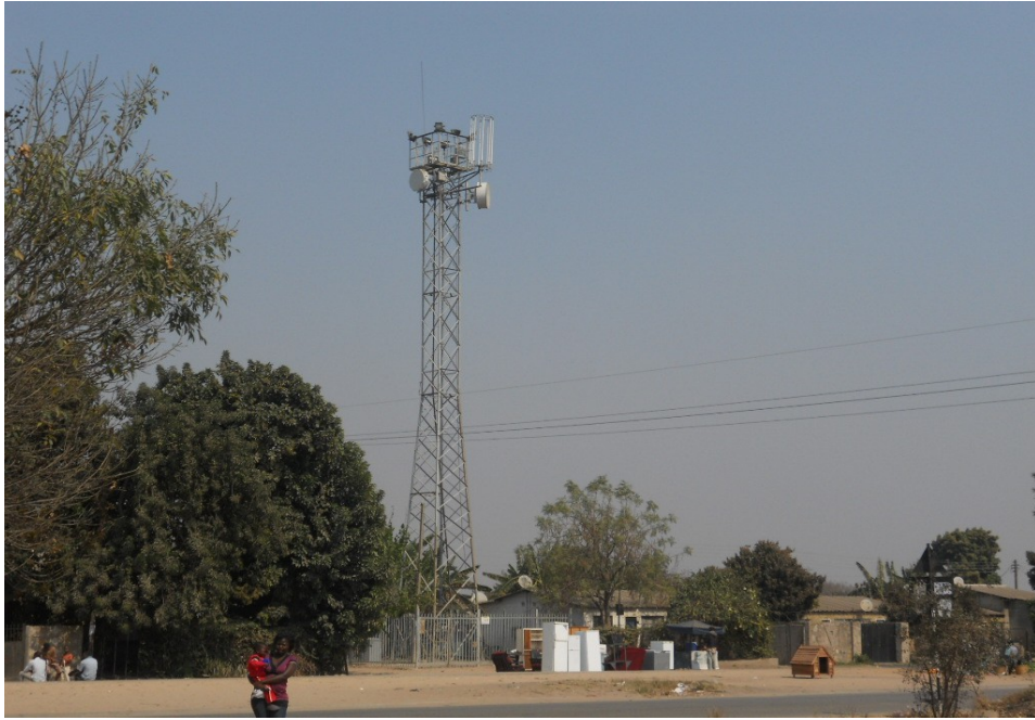
Tower light converted to a base station.
