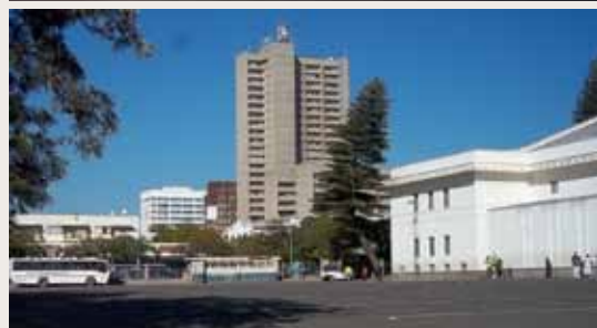
Bulawayo City Hall Car Park.
